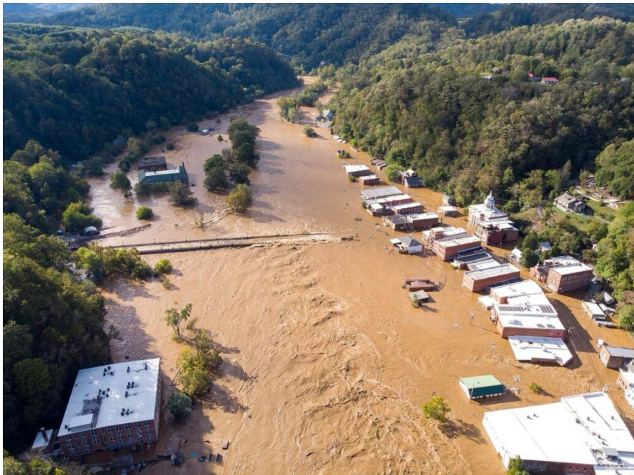
Flooding in downtown Marshall (Old Marshall Jail Hotel)
