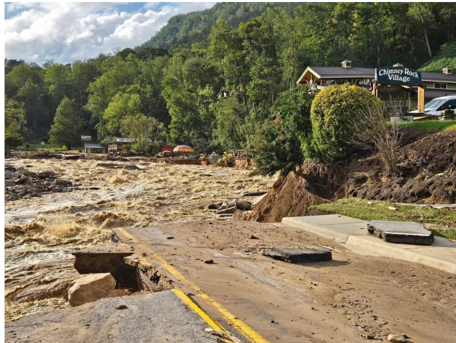
Flooding and damage in Chimney Rock (Vernon Turner)
