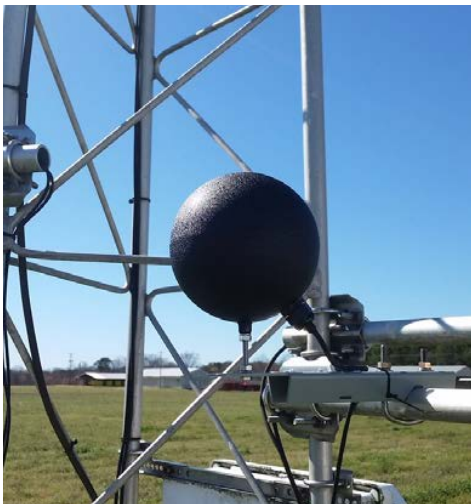
This black globe thermometer was installed at the Rocky Mount ECONet tower on March 3, 2018.
