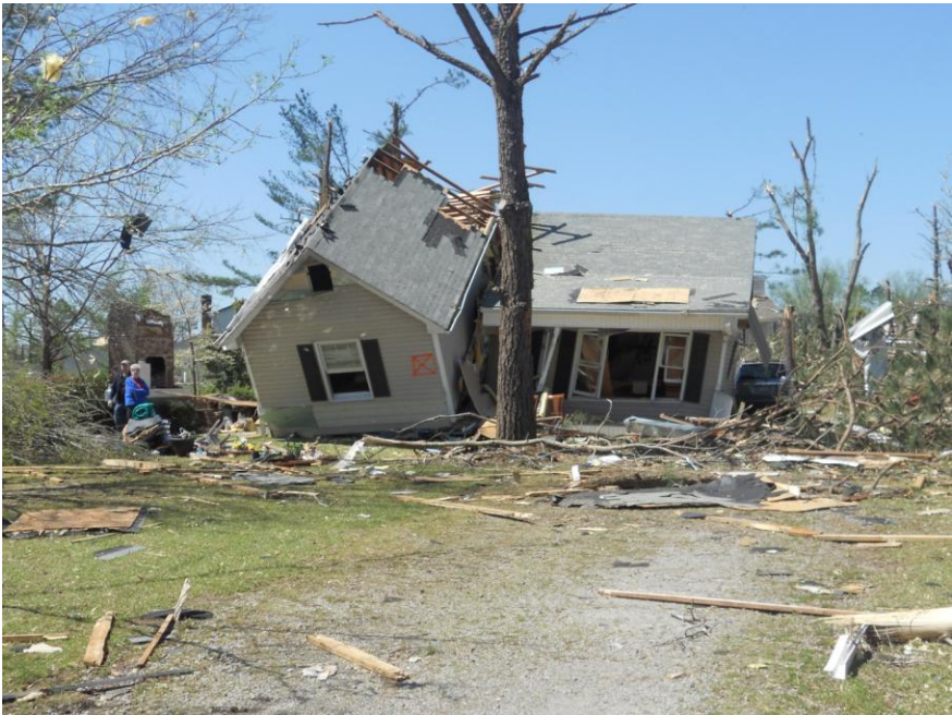
Photo 2 (Residential damage in the St. Andrews subdivision in Sanford)
