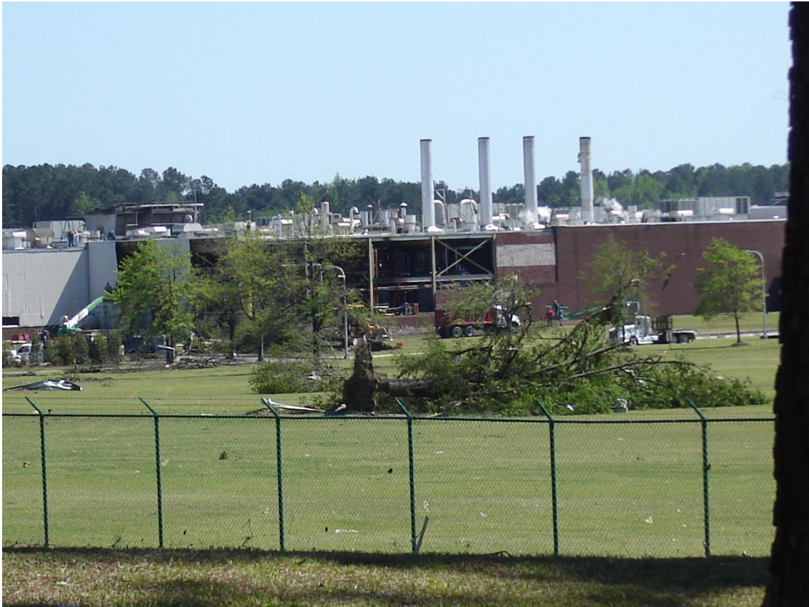
Goodyear plant along highway 401, northern Cumberland County, NC.
